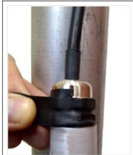
Figure 23: Applying sealant tape to an external connection
