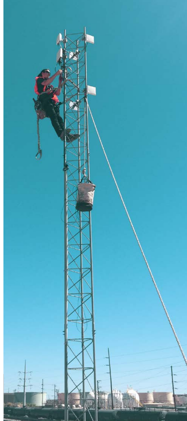
FiberinMotion® base stations deployed along the UTA tracks
